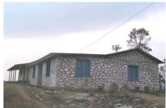
Office building of Janakalyan
