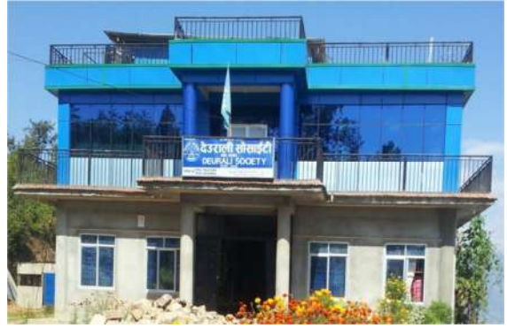
10.3 Office cum Resource centre building under construction
